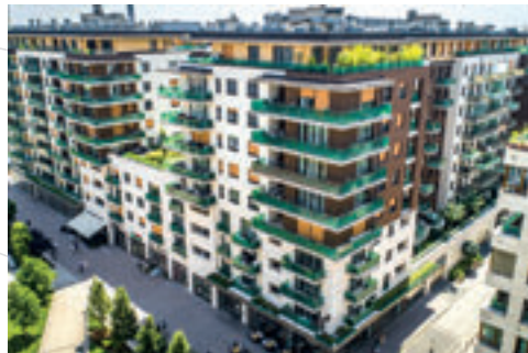
Cordia Park Residence 1, 2 474 homes
